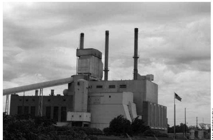
James DeYoung coal fired power plant in Holland.
